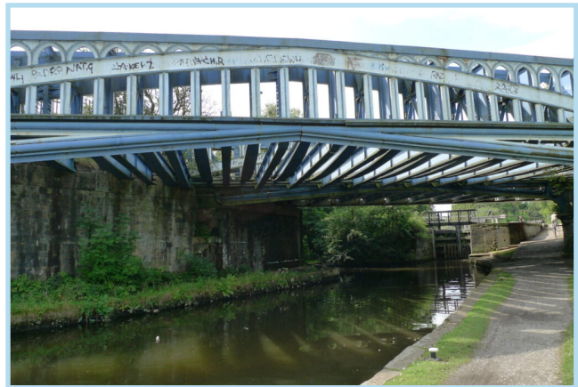
Railway Bridge over the Rochdale canal
